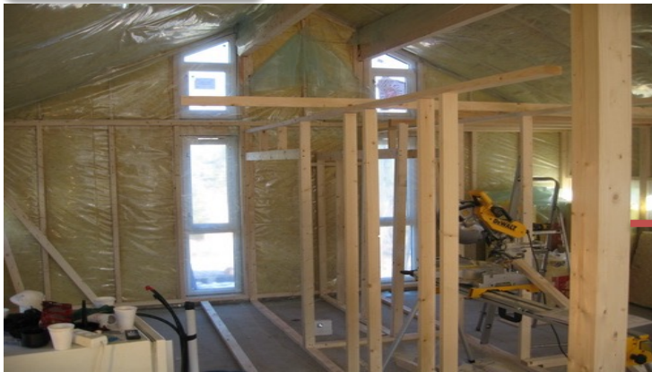
Building structure finished, Inside work on track
