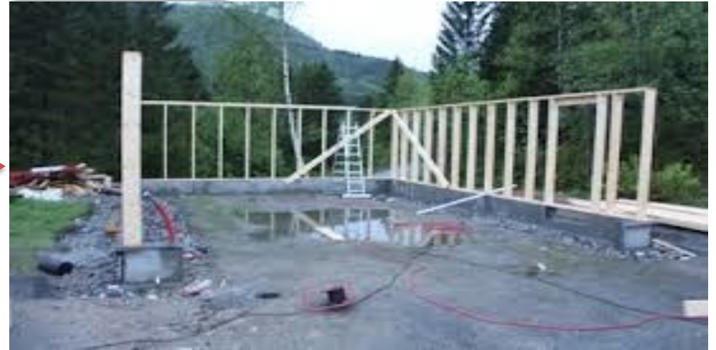
Foundation finished, building structure started A "proof" that you can do it, PoC (Proof of Concept)
